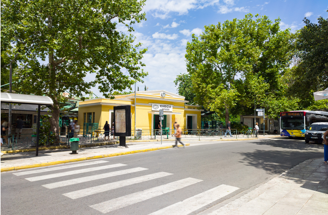
Kifissia ISAP train station
